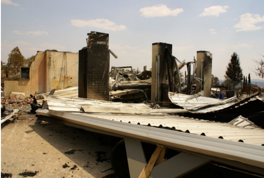
Destroyed buildings in Eden-Monaro.
